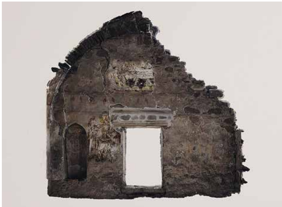
Fig. 11. a – 3D model of the west interior wall of St. Petka's rendered in 3DS Max; b – Rendered 3D model of the west interior wall with colour decorrelation applied
