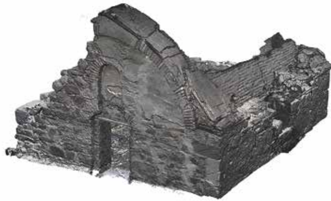
Fig. 6. Medium density, coloured point cloud of the St. Petka Church
