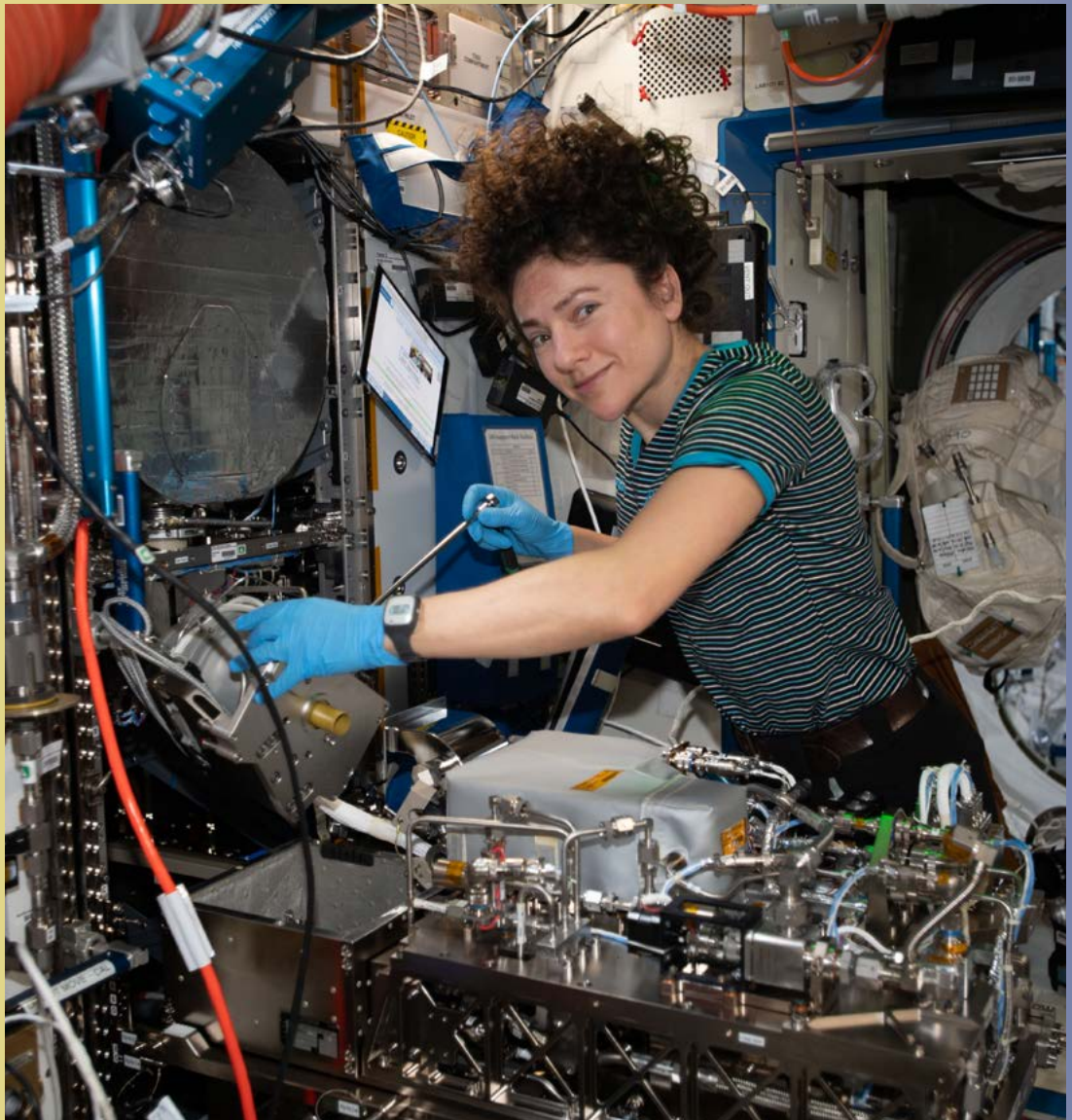
Expedition 62 flight engineer and NASA astronaut Jessica Meir works on orbital plumbing tasks inside the International Space Station Tranquility module's Life Support Rack in February of 2020. Credit: NASA
