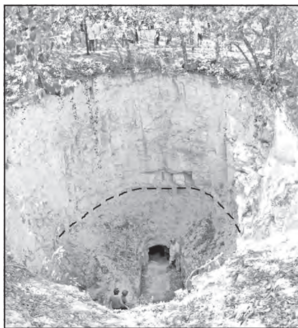
Figure 3: Entrance sinkhole after completion of the project during the open house. The former level of the sinkhole is indicated by the dashed line.
