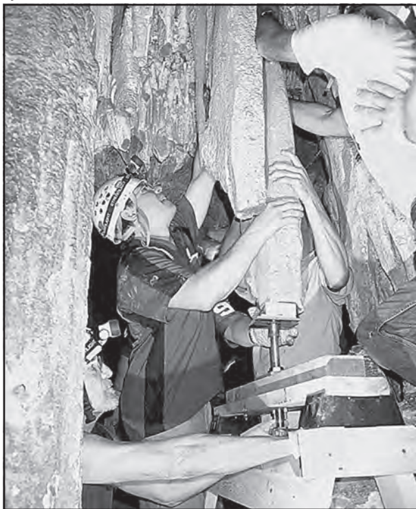
Figure 5: Dennis Hoberg and others position the large stalactite while Jim Werker adjusts the screw jack support structure. Photo by Val Hildreth-Werker.
