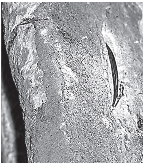
Figure 7: To reinforce the pin and epoxy repair, stainless steel wire is threaded through small drill holes above and below the upper break-joint. Alongside the wire, there are additional stainless pins installed at an angle up through the break-joint and into the ceiling.
