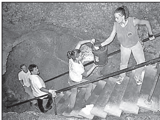
Figure 2: In the Caverns of Sonora (Texas, USA), cave restoration science goes hand-in-hand with willing caver workers, as shown in this of a chain of cavers passing buckets up the stairs. (Photo by George Veni.)
