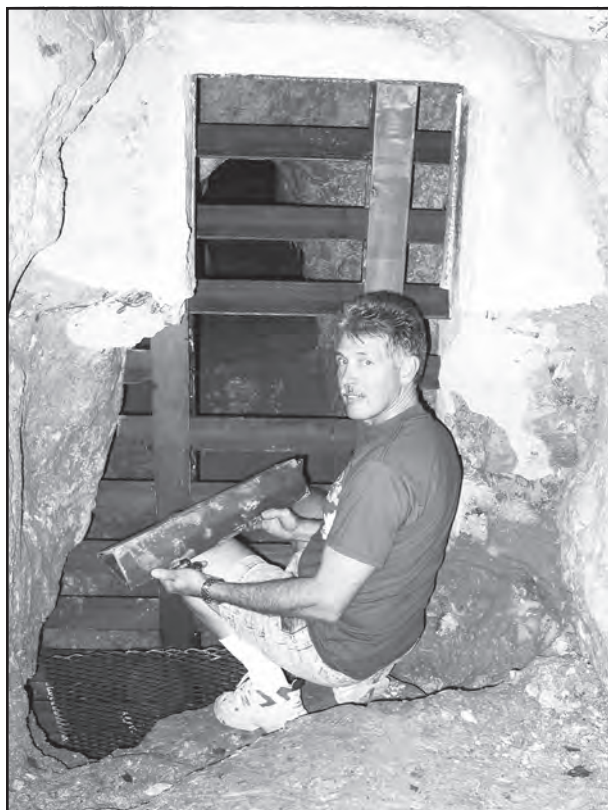
Figure 4: New entrance gate which allows unobstructed flow of nutrients, water, and air.
