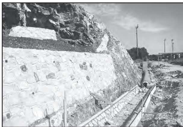
Figure 1: Construction of motorway. Representation of cave, rock scarps, and tubes for water collection from road.
