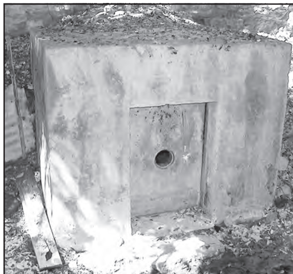
Figure 1: Old bunker entrance gate prior to start of the restoration project.
