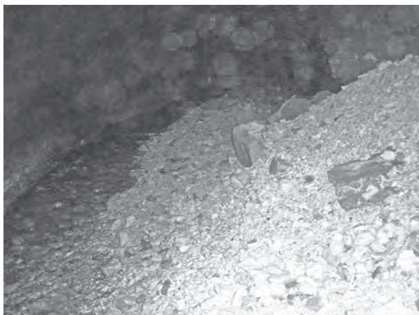
Figure 5: A previous bulldozer track transformed by winter flood waters into an amorphous rubble mound that may reach 2 meters in thickness downstream from the shaft.
