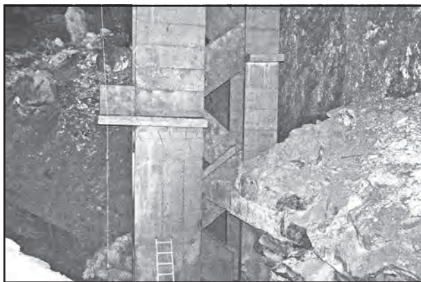
Figure 4: Accumulated construction rubble on natural ledges to the east (top left) and west (right) of the stairway.
