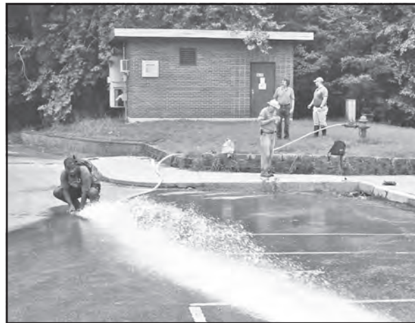
Figure 2: Tennessee State University students test the parking lot filter system in preparation for a larger project looking at parking lot runoff around the Mammoth Cave Historic Entrance.
