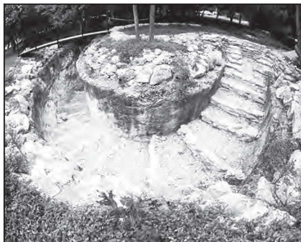
Figure 5: Steps in the trench lead down into the sinkhole under the bridge at upper left.
